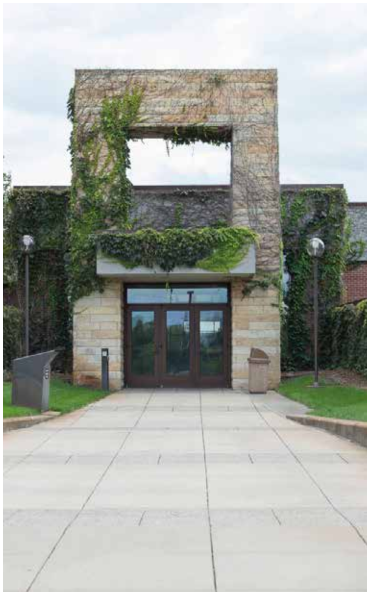
PHOTO BY SUHAIB HAMMAD Main entrance to Coon Rapids
